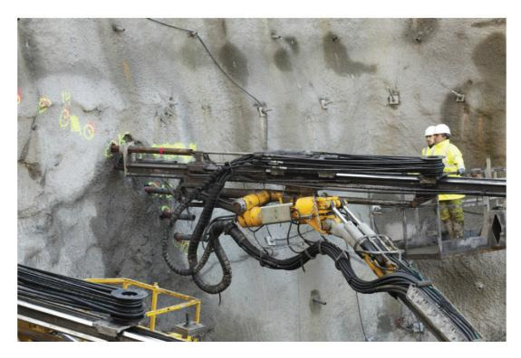
5. Add the extension casings until you reach the desire hole depth (repeat the same process as mentioned on the point 4).
