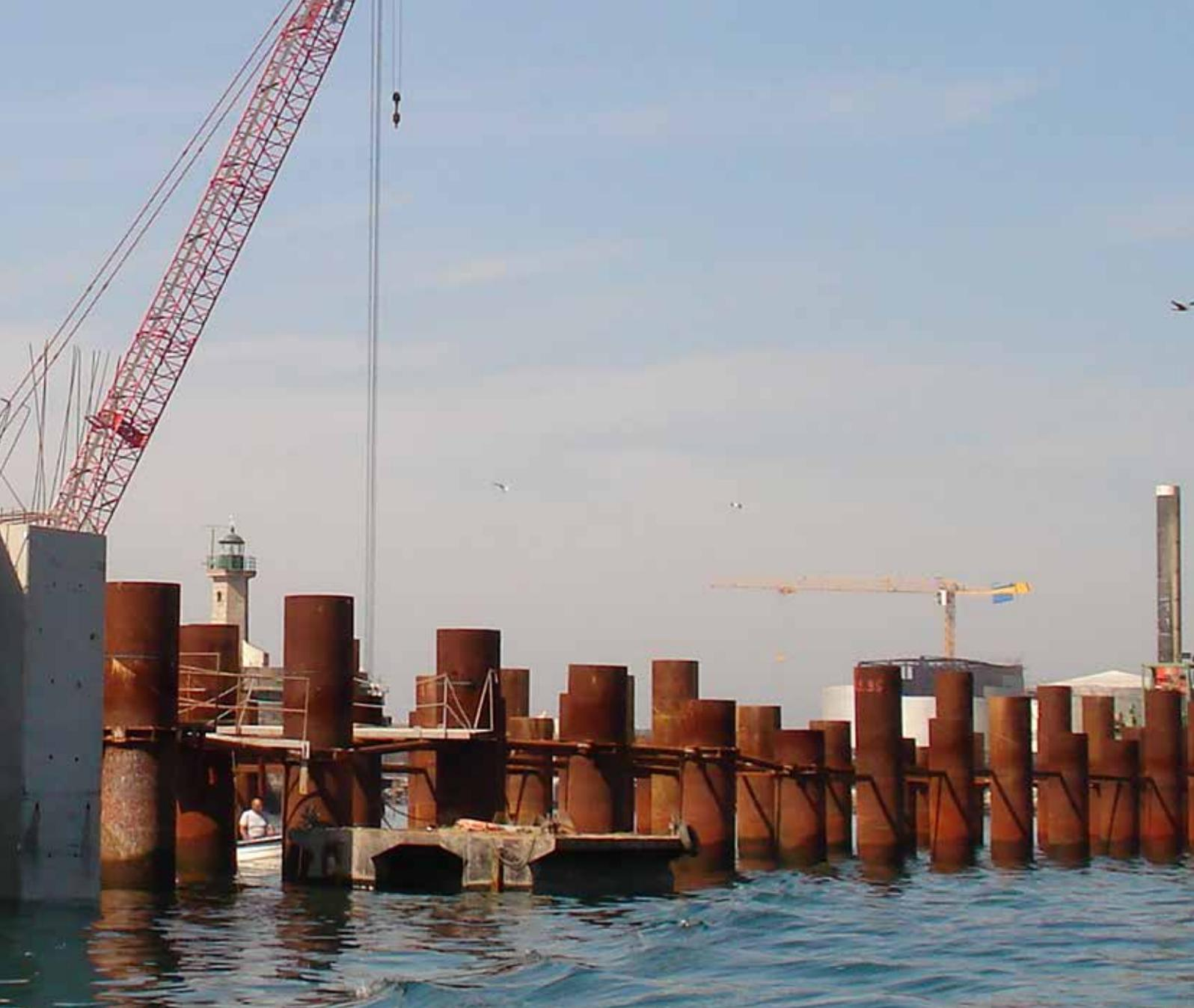
“Casing advancement with DTH hammers is a good method, especially here in Scandinavia where we have to drill through very tough, hard rock or boulders. We use it for installing 219mm–1 220mm casings and it means that we can drill in every type of ground with good accuracy. I was particularly surprised at the good performance of the hammer in the new system which, even in our Finnish hard rock, gave excellent penetration.”
