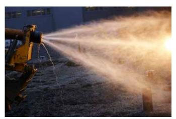
A conventional DTH drilling system directs the compressed air from the flushing grooves straight into the ground with a high intensity, causing the air to rapidly spread to surrounding foundations.
