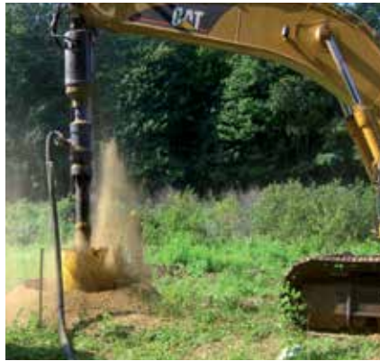
Backhoe with rotary head
