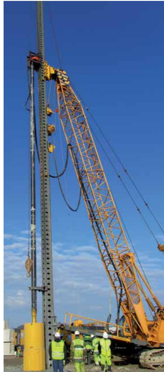
Top drive with centralizer
