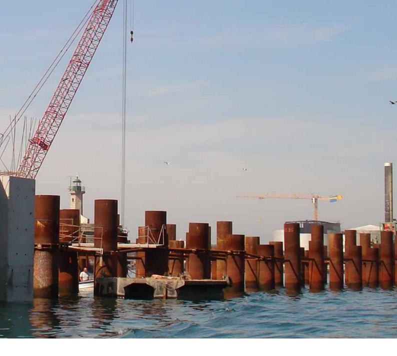
"Casing advancement with DTH hammers is a good method, especially here in Scandinavia where we have to drill through very tough, hard rock or boulders. We use it for installing 219mm—1 220mm casings and it means that we can drill in every type of ground with good accuracy. I was particularly surprised at the good performance of the hammer in the new system which, even in our Finnish hard rock, gave excellent penetration."
