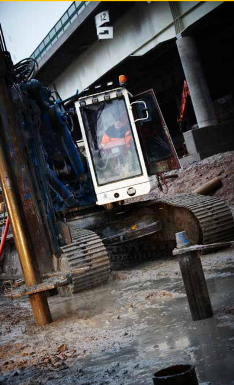
Above: Piling with the Elemex system next to the old bridge.
