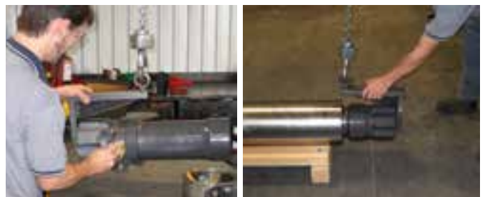
Lubrication and installation of the piston.
